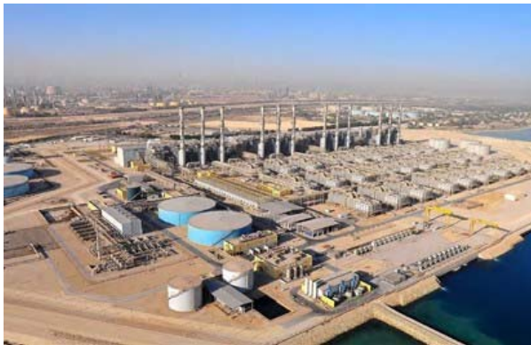
Al Jubail Desalination Plant, Saudi Arabia. Photo: acciona.com
